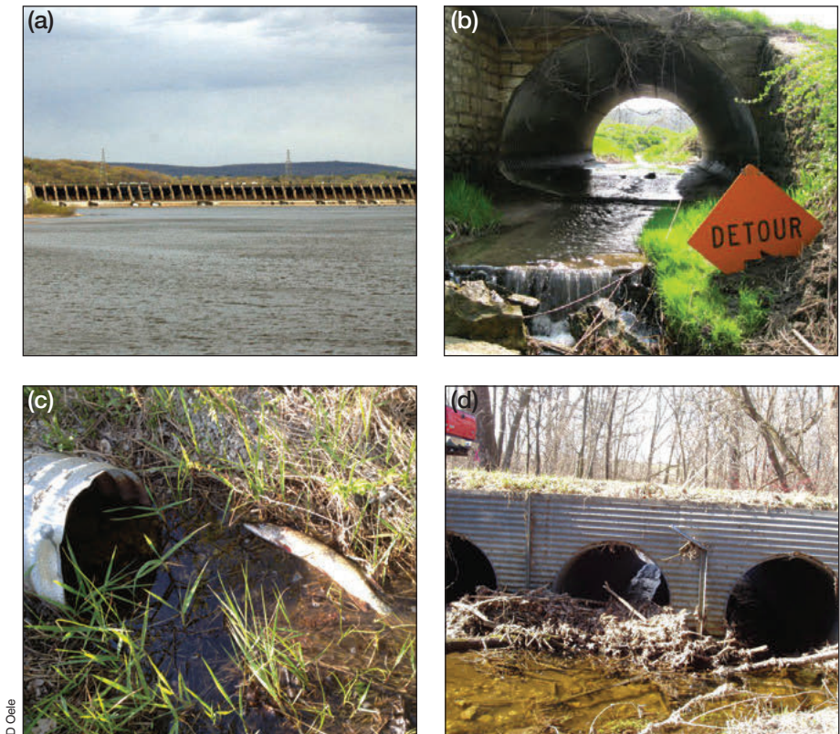
Figure 1. Restoring connectivity between aquatic ecosystems is a global conservation priority. Connectivity between aquatic ecosystems can be enhanced by remediating barriers such as (a) dams and (b) road crossings. These barriers can (c) prevent fish from reaching high-quality breeding habitat, as well as inhibit the movement of (d) nutrients and other material.
